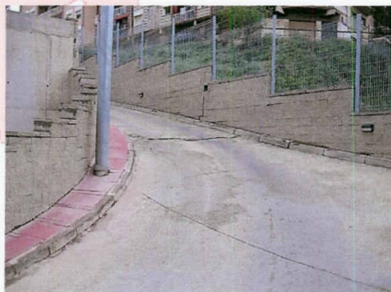
Paviment revolt rampa
